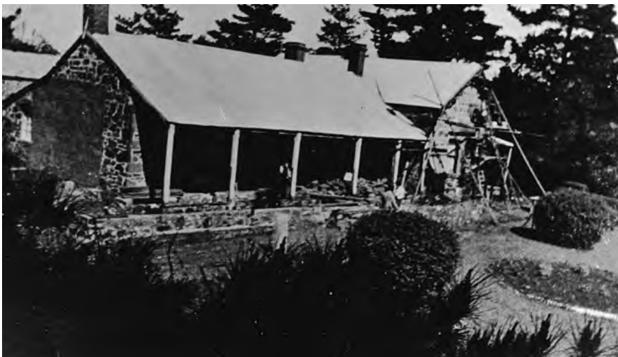
Renovations at Myalla Homestead. Photograph by courtesy of J. Litchfield
