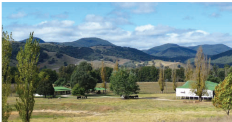
Wee Jasper Station shearers quarters and shearing shed, built by Morris Kershaw around 1940.
